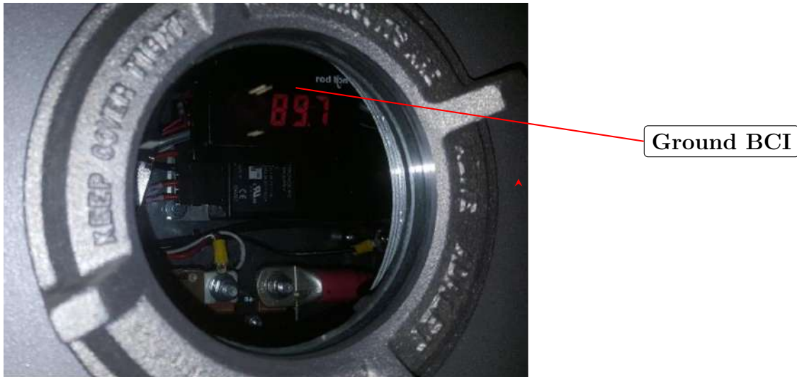
Figure 7.2: Ground Battery Condition Indicator (BCI)
