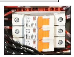
The control system includes circuit breakers in place of glass fuses. The circuit breakers can be easily reset if a problem occurs.
